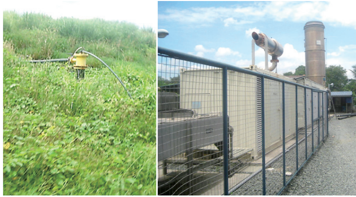
Photos: Methane is generated from the anaerobic decomposition of organics in SWDS. While avoidance may be achieved through waste diversion, methane from existing SWDS may be captured, flared, and/or utilized such as this methane-to-electricity project in Quezon City.
