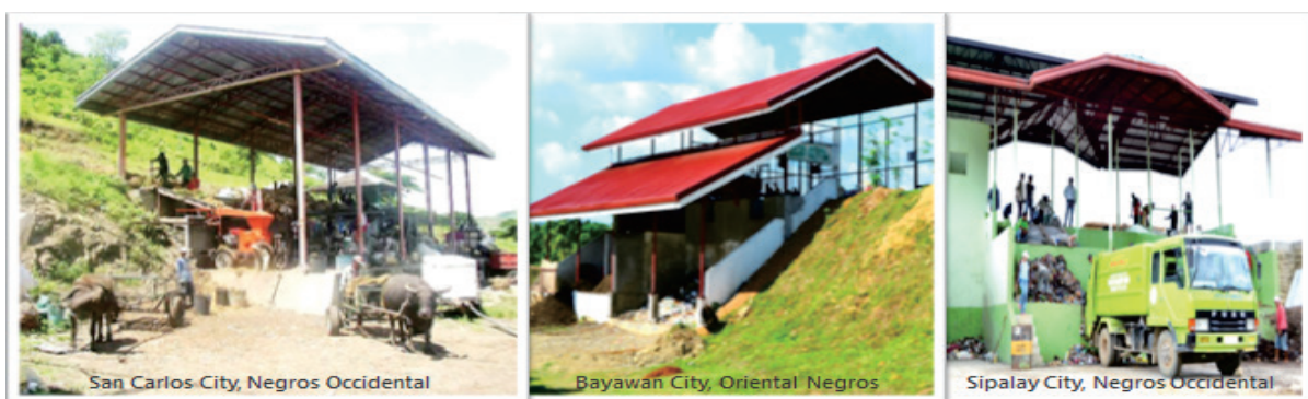
Photos: Centralized gravity-driven MRFs are built in the Integrated Eco-Centers in Negros Island [Acosta, et al., 2013]
